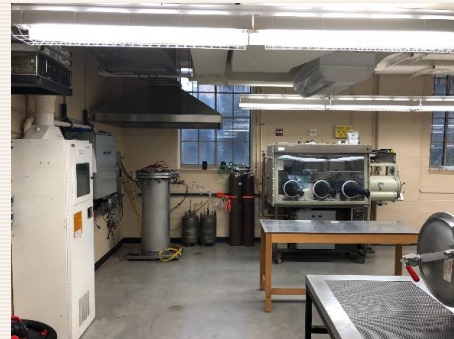
HTF purification and manufacturing system
