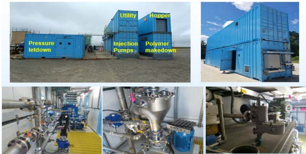
Figure 7: Polymer injection unit on the J-pad at Milne Point.
