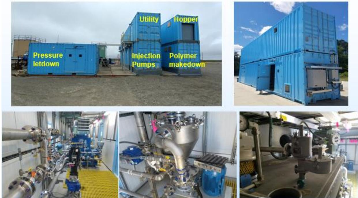
Figure 6. Polymer slicing unit (source: SNF)
