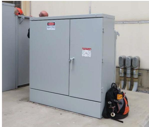
**Photo 3.1.2.1: Installation of new transformer (right) replacing old transformer (left).**
