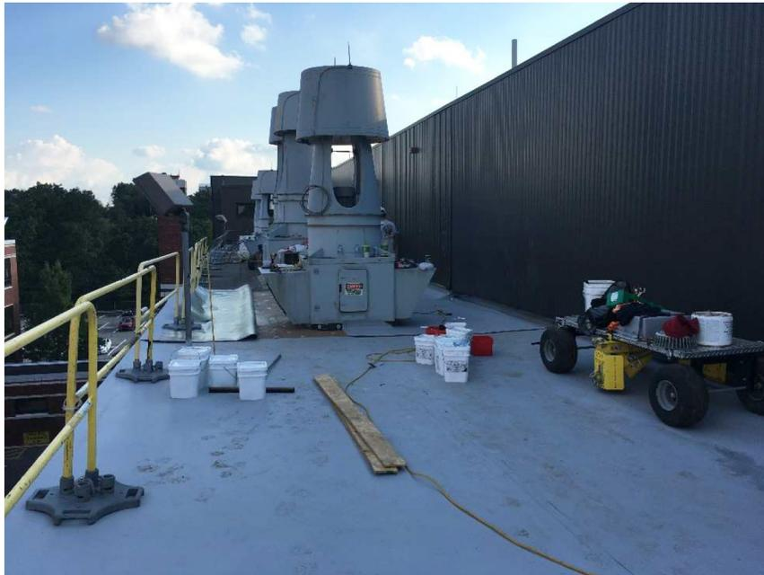
Photo 3.2.2.1: B-84 Roof Replacement – New roof in foreground, old roof in background.
