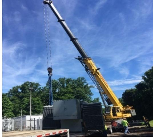
**Photo 3.1.2.2: Installation of new transformer (right) replacing old transformer (left).**
