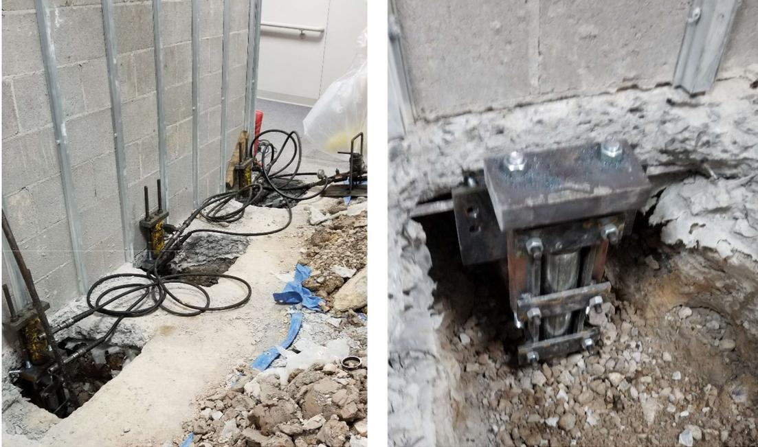
Photo 3.1.2.6: Building 26 Foundation Repair.
