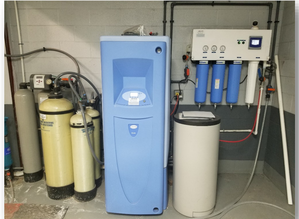
Deionized Water System
