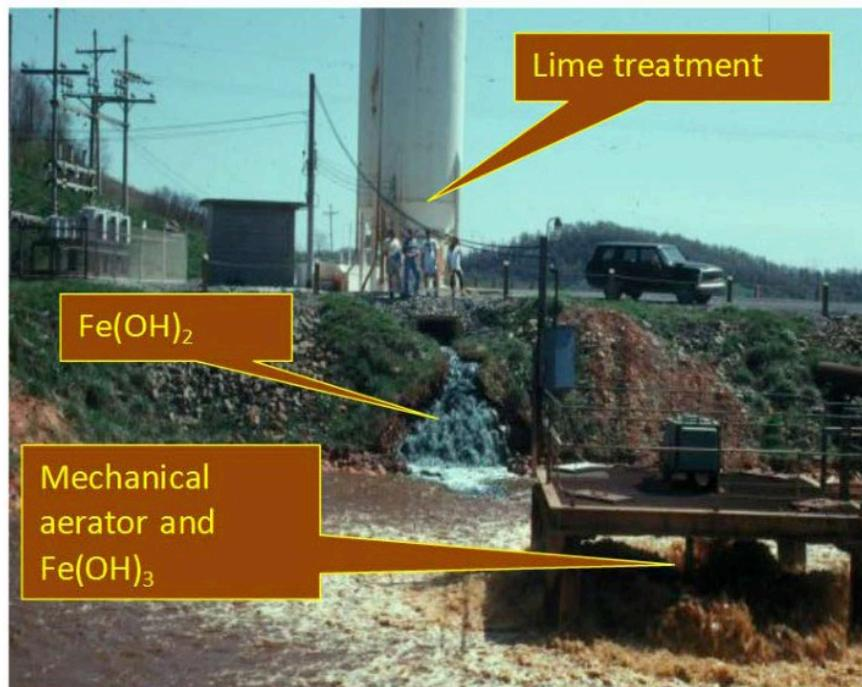
Typical AMD treatment facility showing the lime treatment unit, reduced  $\text{Fe}(\text{OH})_2$  sludge (blue), the mechanical aerator, and resulting  $\text{Fe}(\text{OH})_3$  oxidized sludge.
