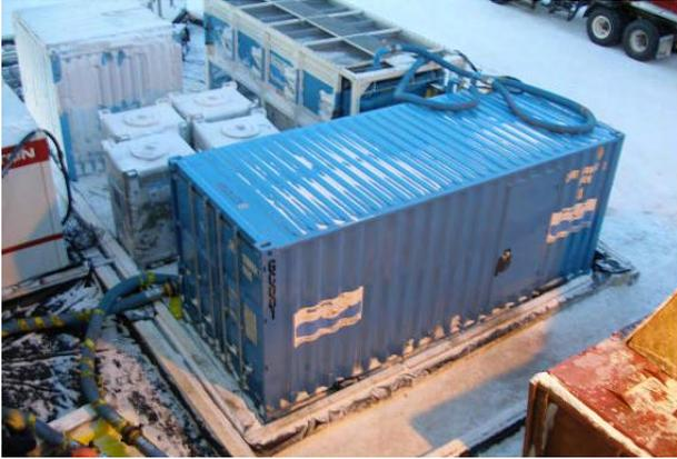
Figure 7: DrillCool, Inc. Heat Exchange Mud Chilling Unit onsite at Mount Elbert-01 Ice Pad.
