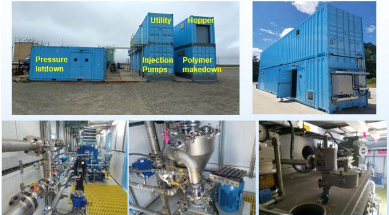
Figure 11 Polymer injection unit on the J-pad.
