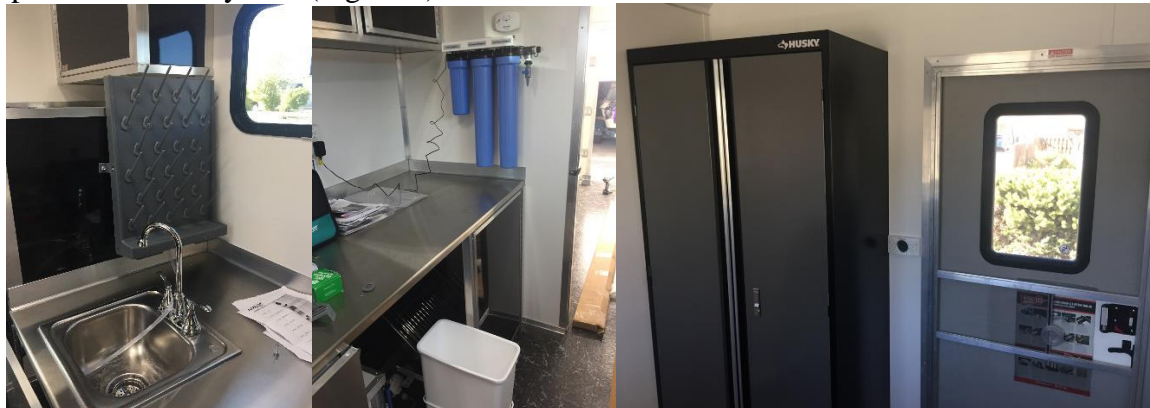
Figure 4. Images of the build-out of the mobile operations center. Left: drying rack for laboratory glassware, middle: ion exchange water treatment system, right: storage cabinet attached to wall.
