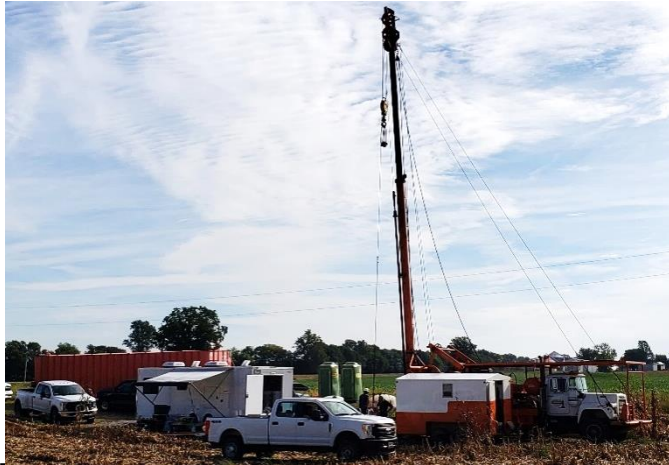
Figure 2. Field work was conducted at the Rexing #4 well head in September of 2018. A workover rig, the mobile laboratory, and a frac tank filled with 100bbl of fresh water were on site during the field work.
