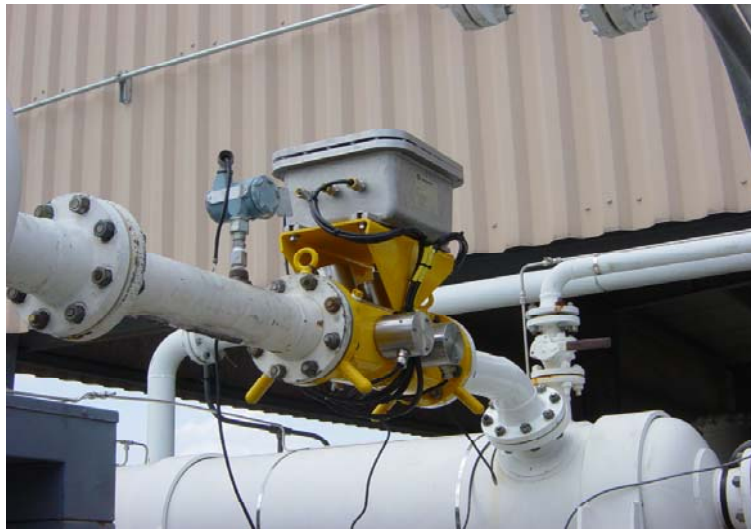
Figure 5-33. 4-inch Instromet Ultrasonic Flow Meter in Suction Choke Tube at ARCT Test Bed
