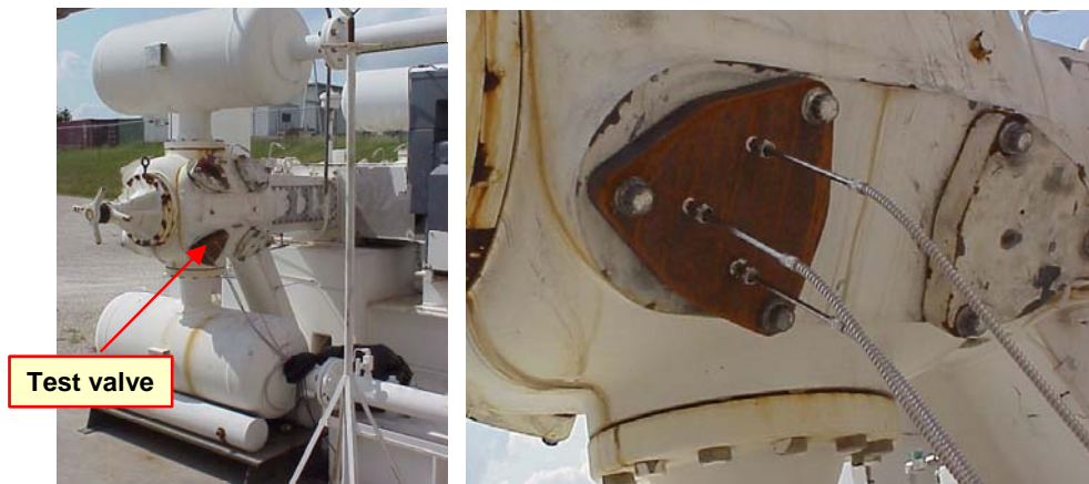
Figure 4-27. Ariel Reciprocating Compressor Used in Measuring Valve Motion (Left) with Optical Position Probes Mounted on Valve (Right)
