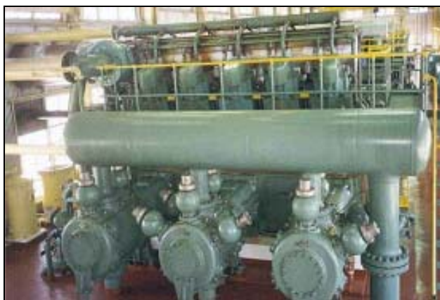
Figure 1-2. Slow-Speed Integral Compression Running at Less Than 300 RPM in the 1,500 to 2,500 HP Range With Pulsation Control Systems
