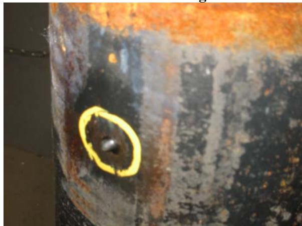
Photo 23: External View with Flex-Plug Extrusion
