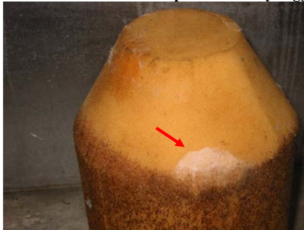
Photo 17: Soft Sealant Lump Removed by Pigging
