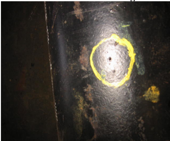
Photo 22: External View before Flex-Plug
