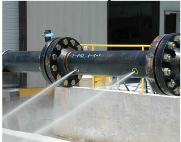
Photo 7: Pinhole Leak Rate Testing
