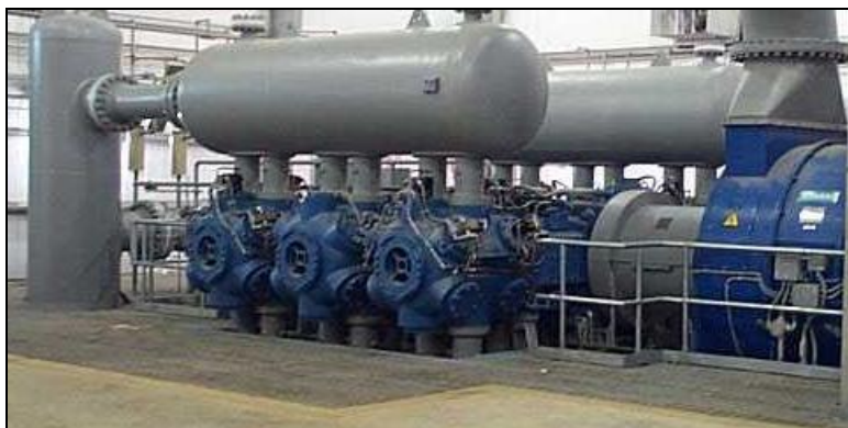
Figure 3. Modern Large High-Speed Separable Compressors Running in the 500 to 1,000 rpm Range in the 8,000 to 10,000 hp Range
