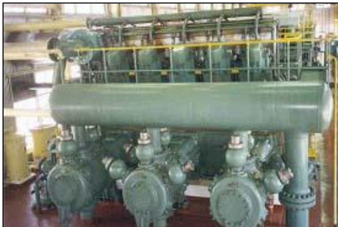
Figure 2. Slow-Speed Integral Compression Running at Less Than 300 rpm in the 1,500 to 2,500 hp Range With Pulsation Control Systems
