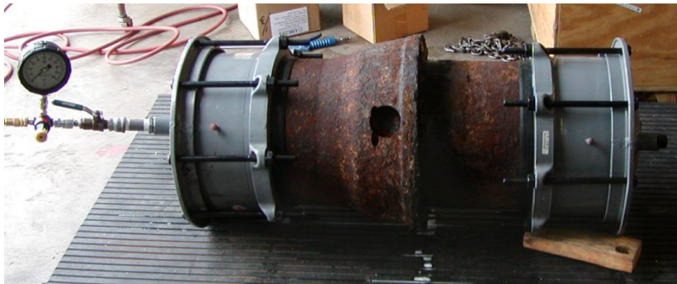
Figure 14. Cast Iron Joint Tested for Leaks
