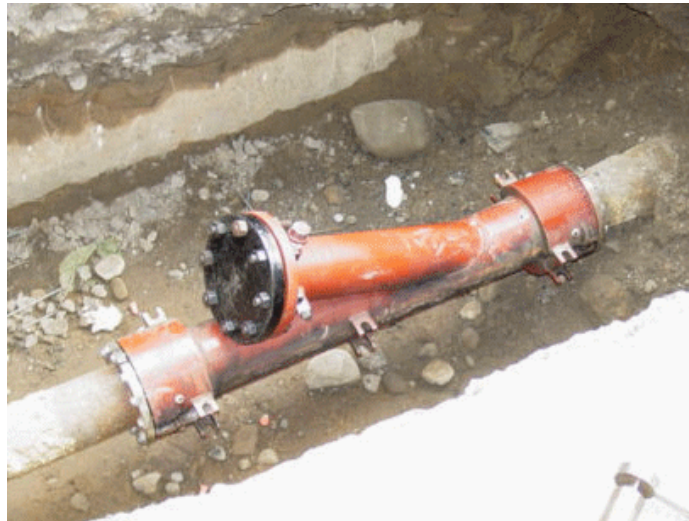
Figure 46. Entry Fitting Ready for Burial
