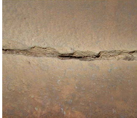
Figure 2. Camera's View of Bell and Spigot Joint Seam
