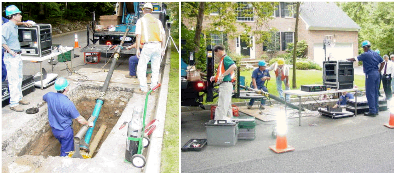
Figure 40. Field Test Site
