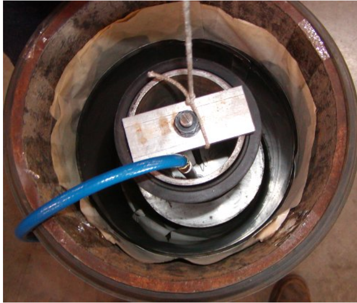
Figure 15. Bladder/Patch Assembly Hung in Joint
