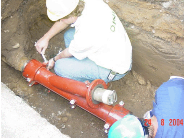
Figure 41. Attaching Entry Fitting to Pipe Prior to Welding
