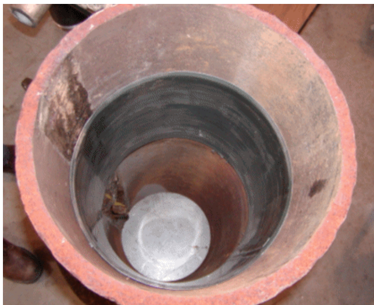
Figure 10. Successfully Installed Repair Sleeve
