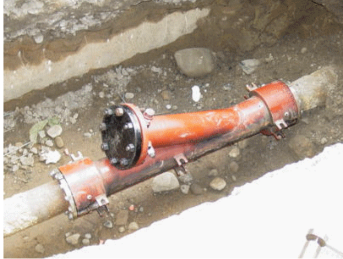
Figure 50. Entry Fitting Ready for Burial
