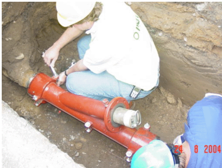
Figure 45. Attaching Entry Fitting to Pipe Prior to Welding
