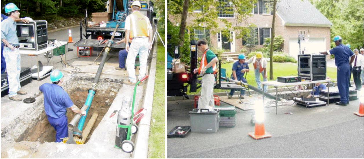
Figure 44. Field Test Site
