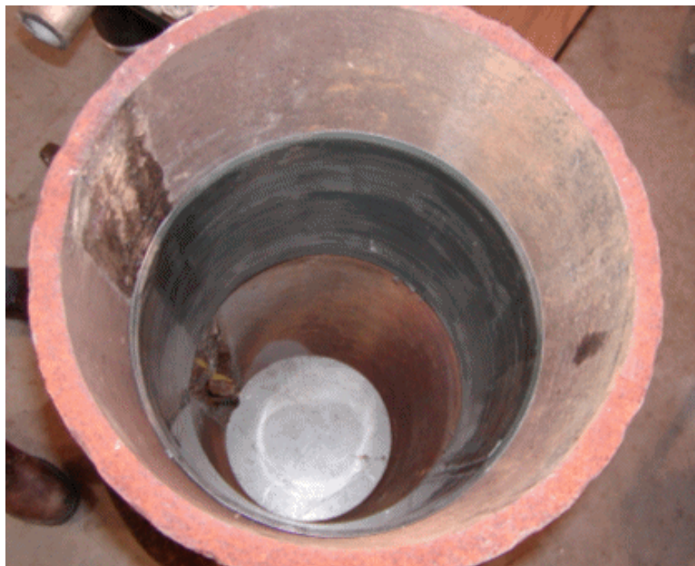
Figure 10. Successfully Installed Repair Sleeve
