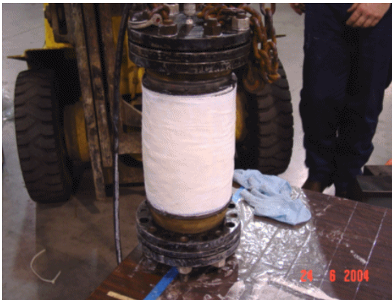
Figure 7. Repair Sleeve with Epoxy Applied
