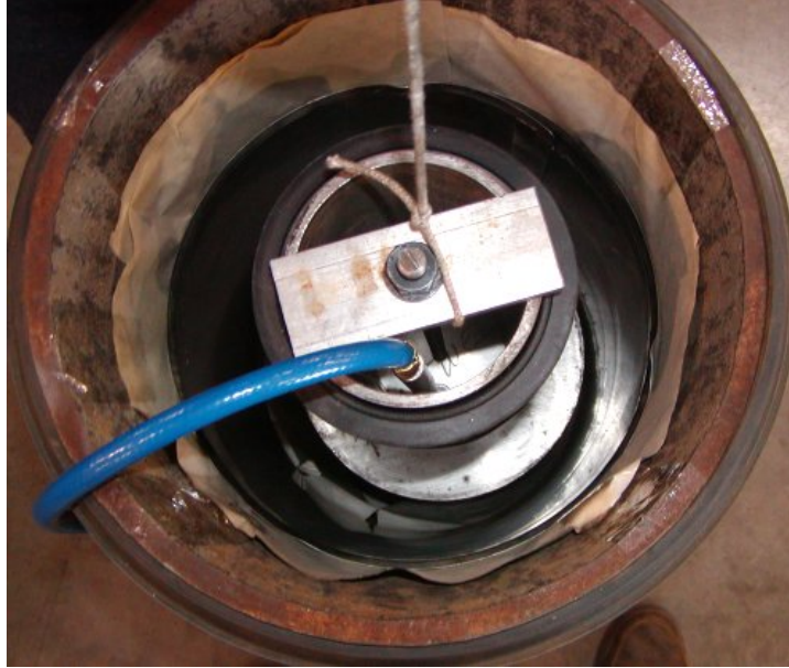
Figure 15. Bladder/Patch Assembly Hung in Joint
