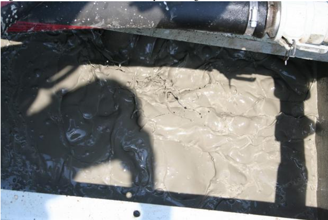
Figure D2: Pre-Stressed Cement slurry in mixing tank
