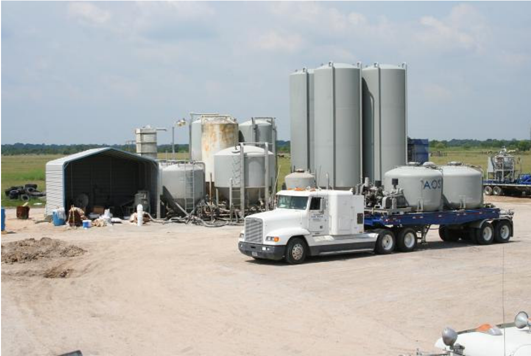
Figure D1: AOS yard facility
