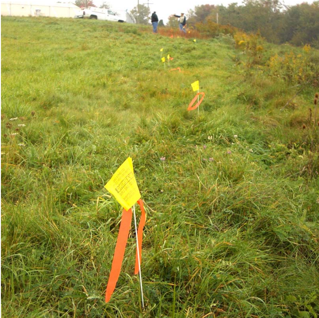
Figure 25: Yellow flags indicate Util-Lite location points. The orange blazes indicate confirmation by an induction locator.
