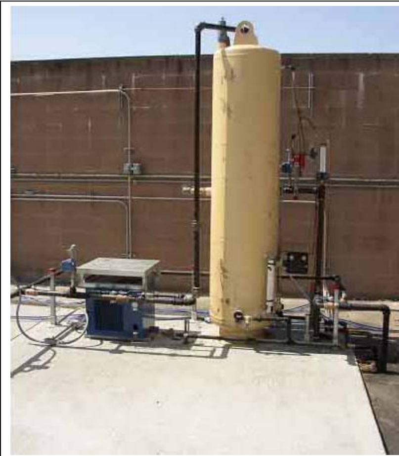
Vertical Free Water Separator with Refrigeration Dryer Unit
