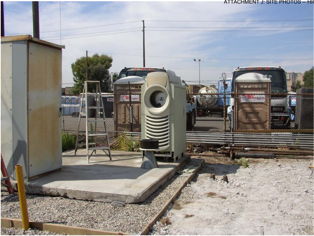
Termo Site During Construction
