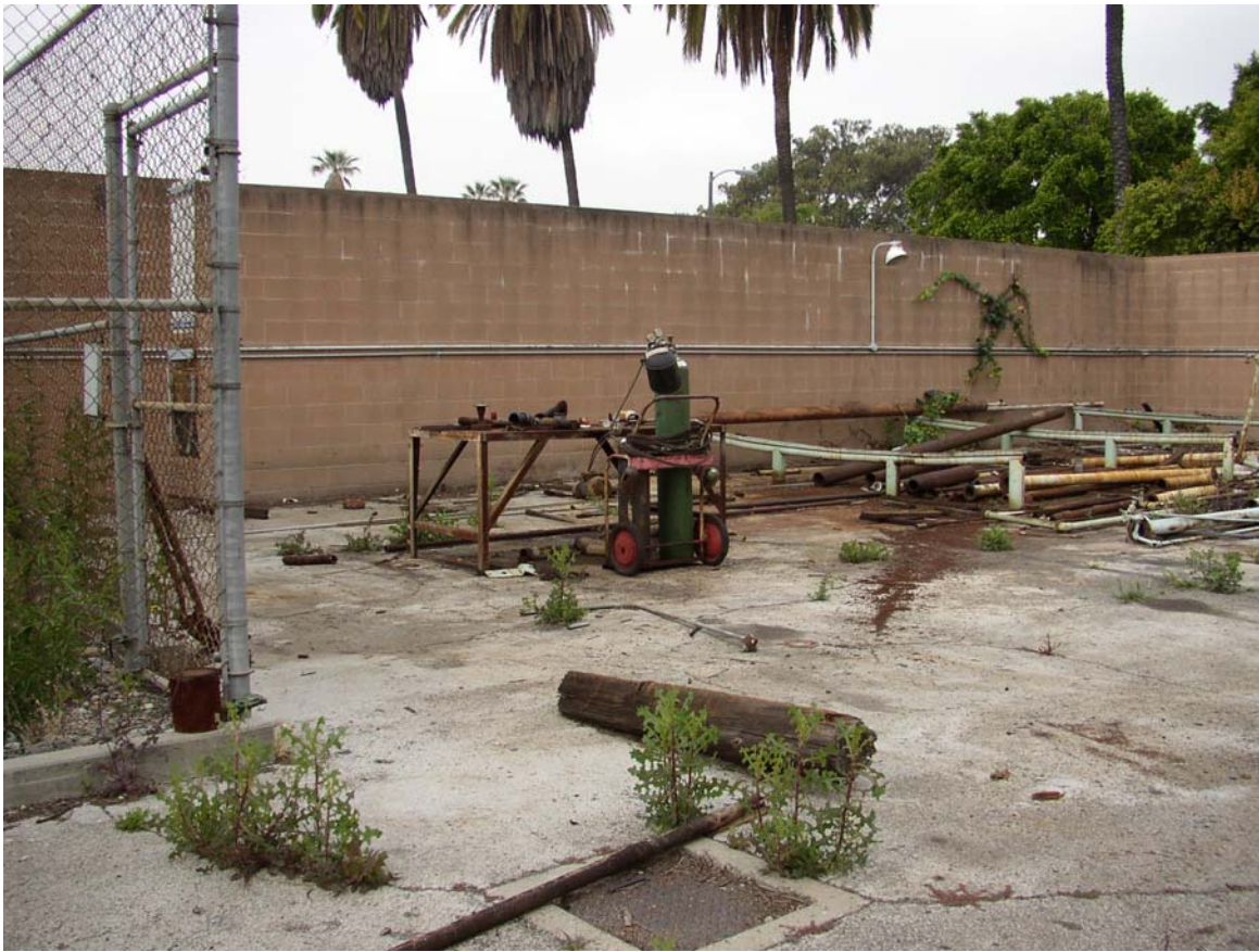
St James site after over 3 years of no production.
