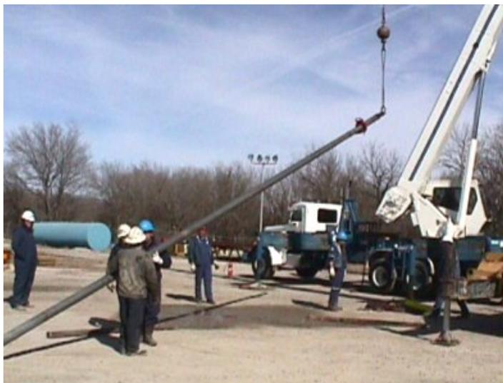
Figure 25. Lifting BHA for Insertion into Well
