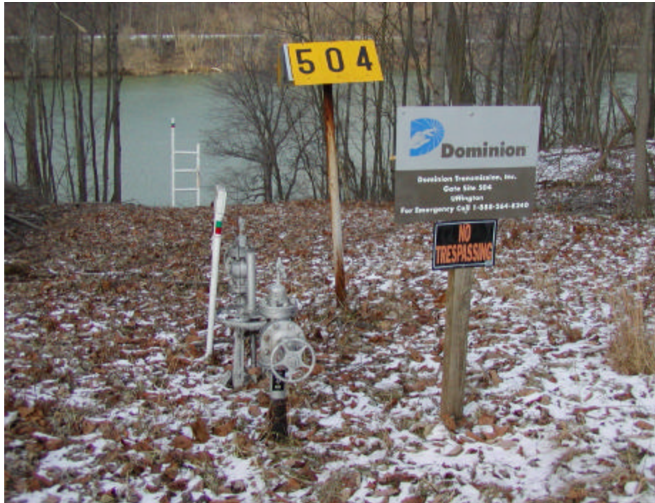
Figure 1: Dominion line 323 near Morgantown, WV, showing the ½" NPT inspection ports on either side of the shut-off valve.
