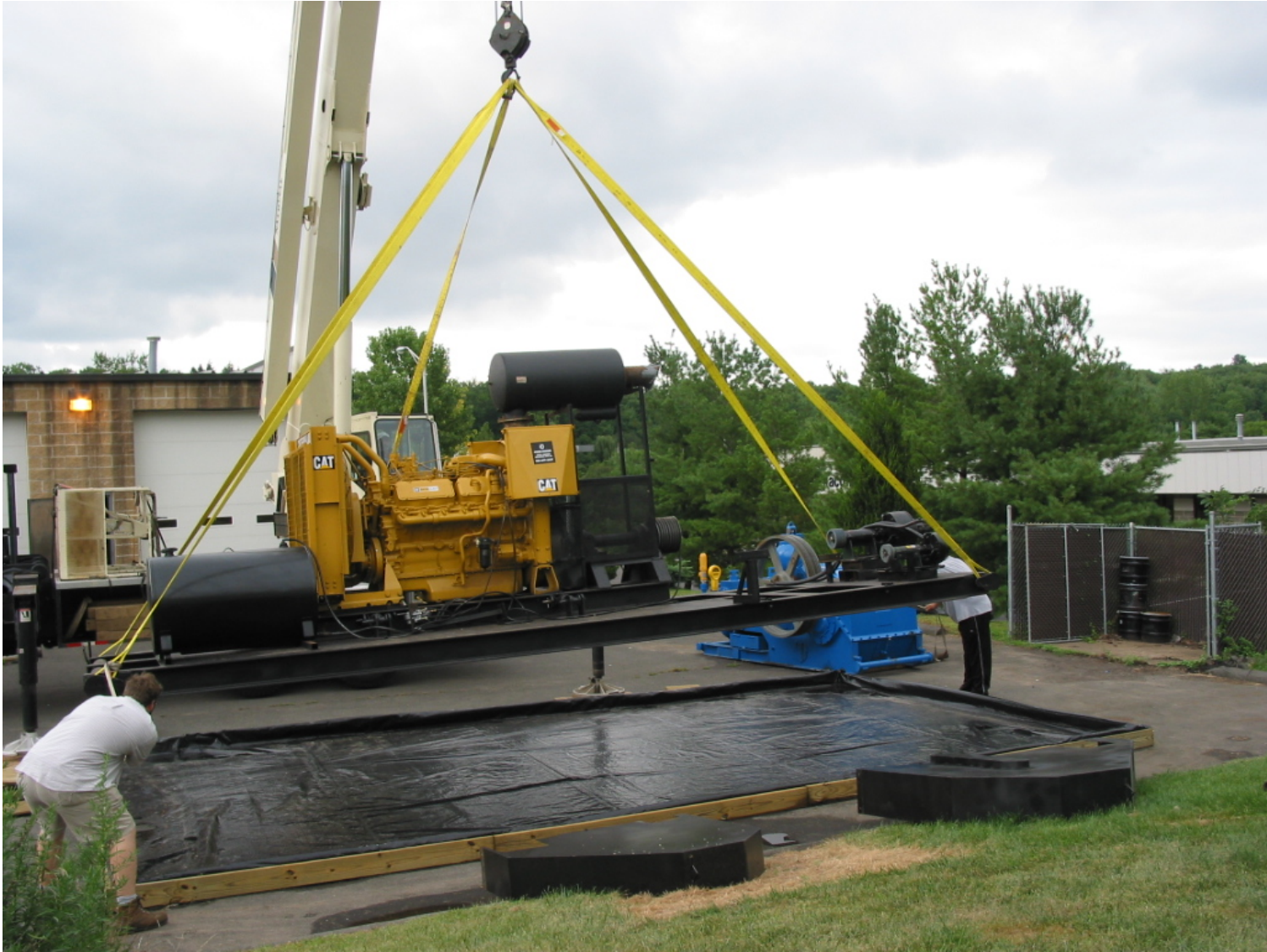
Figure 6: Delivery of motor & frame
