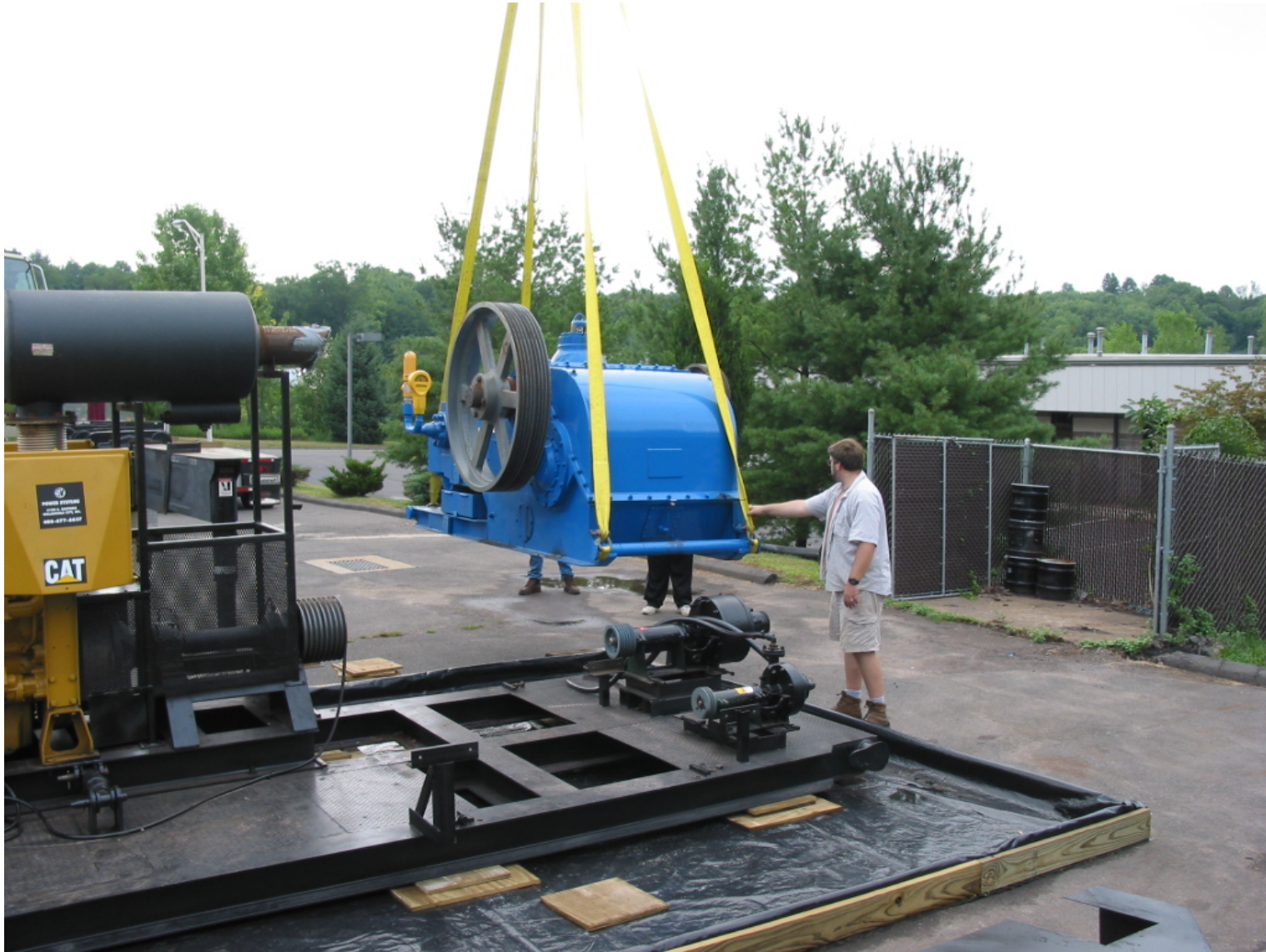
Figure 5: Delivery of pump
