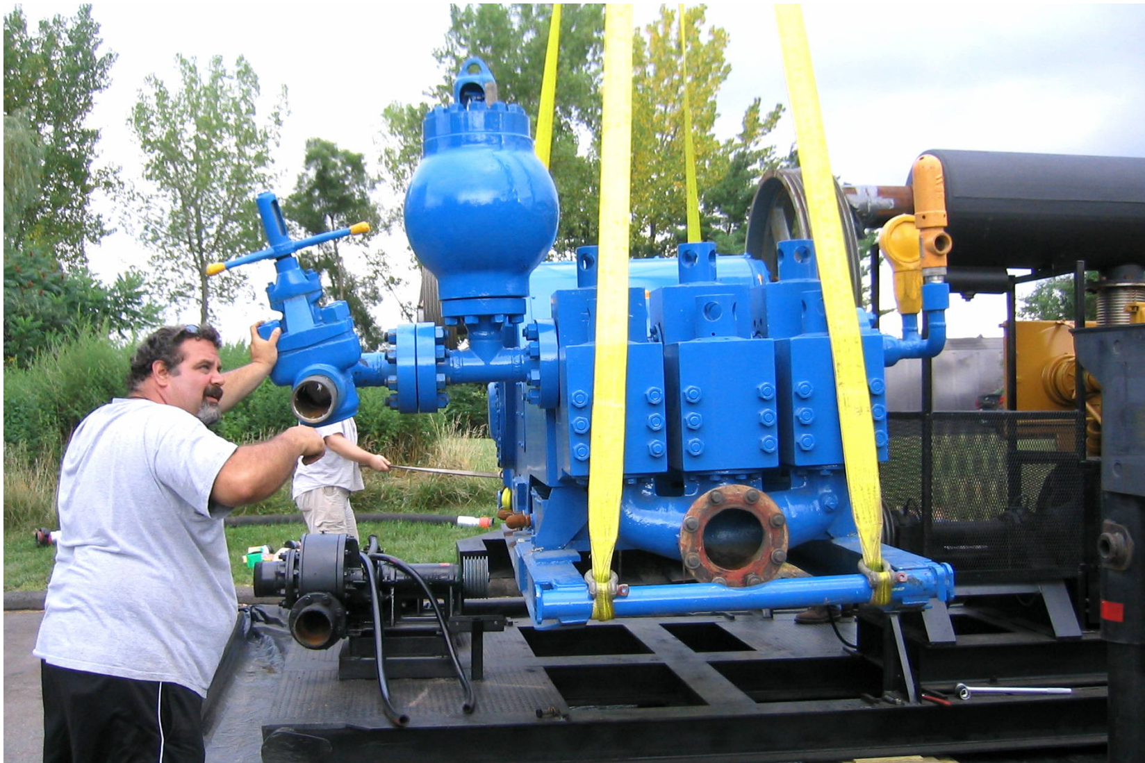
Figure 8: Placement of pump
