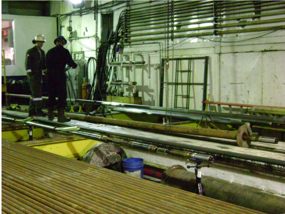
Photo 4: Tractor in Pipe Bay at Nordic 2 Rig Prudhoe Bay, X-30 Well
