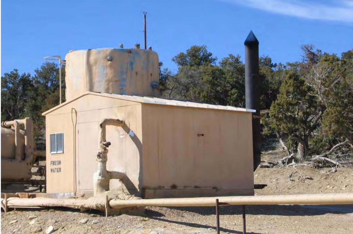
*Figure 14-5. Heat treater with bird screen on the exhaust stack at the El Paso Production Oil and Gas Company Ute Fee 2-33C6, SW1/4SW1/4 section 33, T. 3 S., R. 6 W., UBL&M, in Cedar Rim field.*
