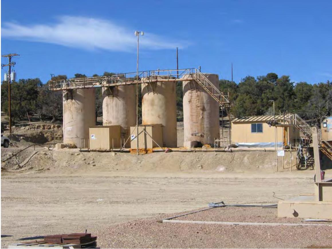
*Figure 14-1. Insulated tanks and heat treater at the Ute Fee 2-33C6 well in Cedar Rim field, SW1/4SW1/4 section 33, T. 3 S., R. 6 W., UBL&M.*
