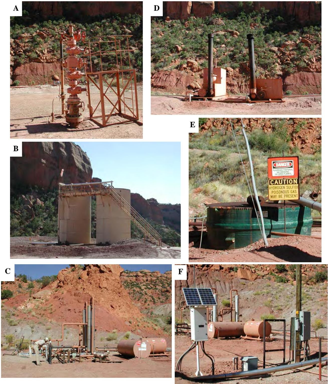
*Figure 15-5. Typical Lisbon well site including: A – wellhead, B - tank batteries, C – dehydrators with chemical storage tank for methanol, D – heated separators (heater/treaters), E – double-walled emergency pit tanks, and F – solar-powered flow meters.*
