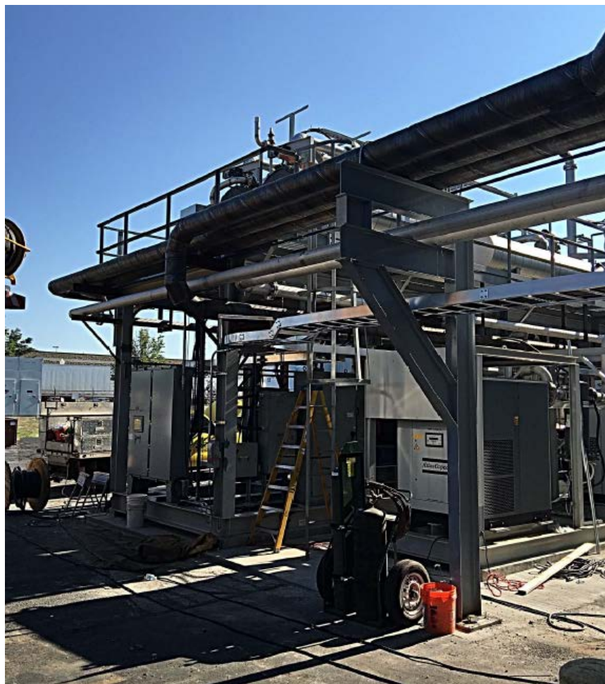
Process and utility lines connected to and from skid
