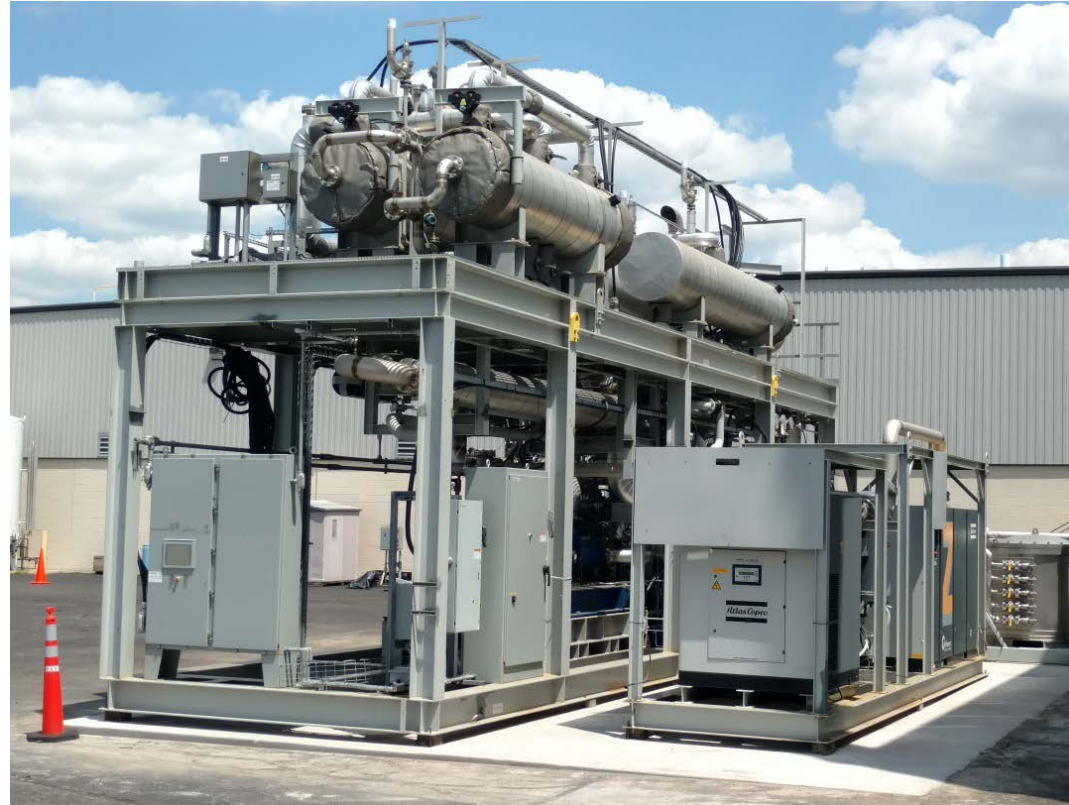
Main skid and smaller low-pressure drop sweep module anchored to foundation
