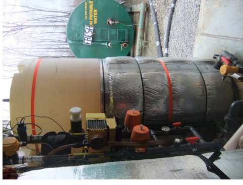
Batch brine recirculation tank
