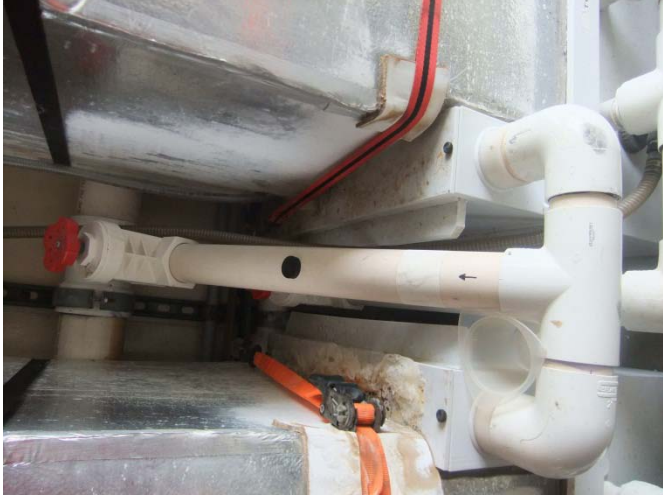
Pipes carrying saturated air from the system and tanks collecting treated water at the side
