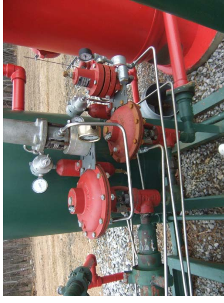
Series of control valves used to reduce pressure before feeding to the production pipeline
