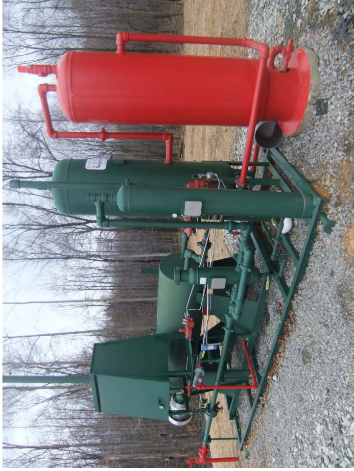
Series of tanks and valves used to reduce pressure and remove water
