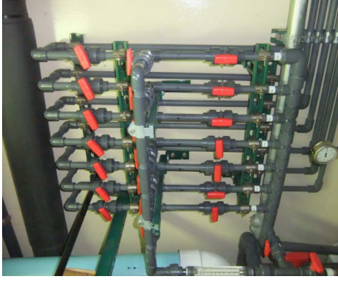
Valves controlling brine flow to treatment towers
