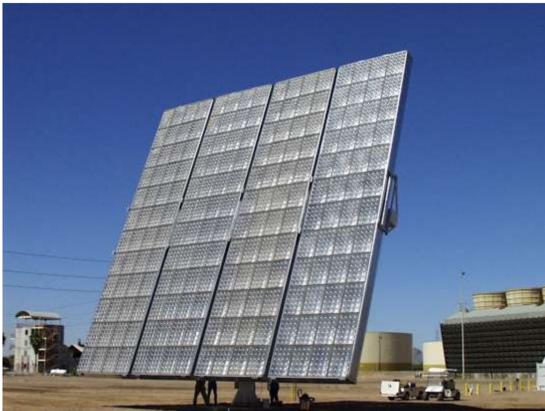
Figure 41: A four MegaModule™ System produces 20,000 watts
