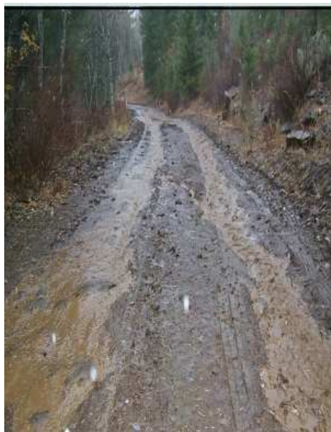
Figure 1. The photograph shows an eroded Forest Service logging road in the National Forest. The challenge is to change the characteristics of forest roads, the principle source of anthropogenic sediment entering streams on Forest Service lands.
