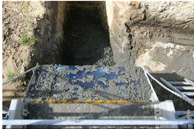
Figure 18 - Mud Pit for Drill Cuttings if needed; The Pit is (3'x 3'x 6')
