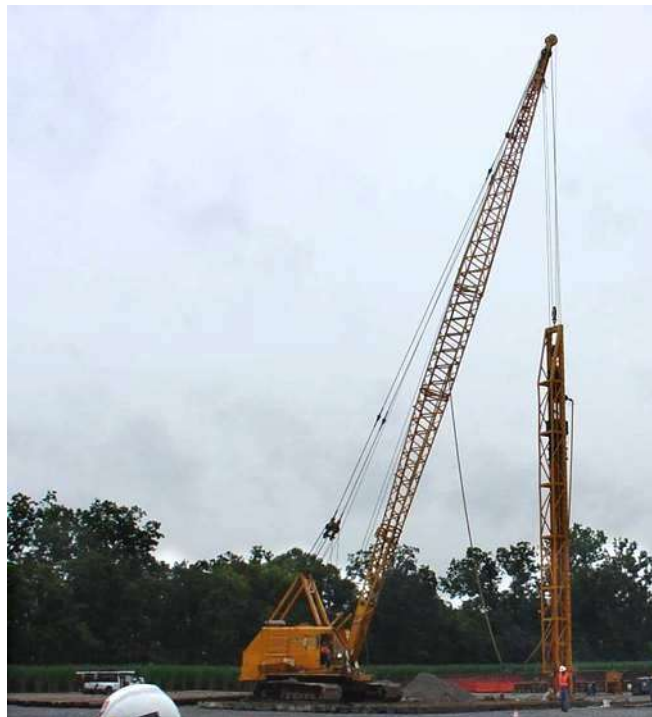
Figure C-8. Pile Driving Operation
