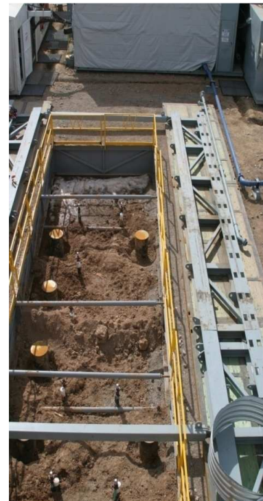
Figure 4. Cellar showing various conductor pipes for wells. Also shown is the rail system for moving the rig.
