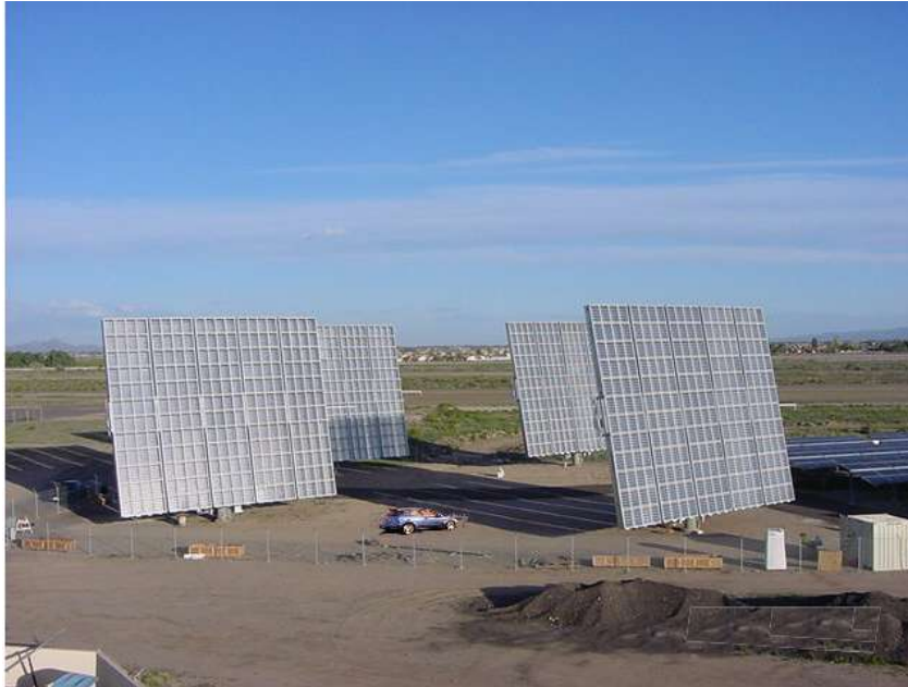
Figure 42: APS's 100 kW Amonix HCPV installation at Glendale, Arizona
