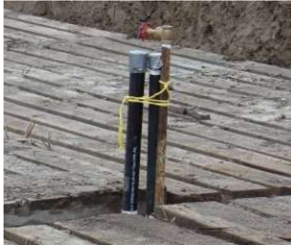
Figure C-6. Water, electrical, and fuel lines for injection package
