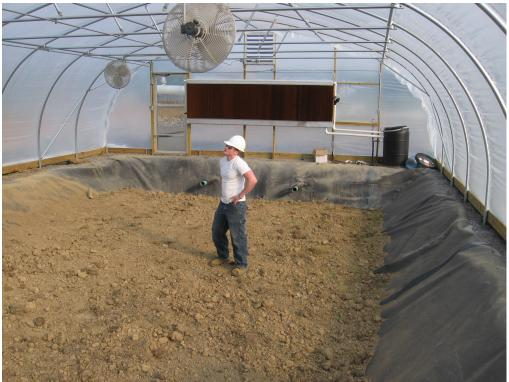
Figure 8. Interior of greenhouse including HDPE liner, hydrosoil and a graduate student.
