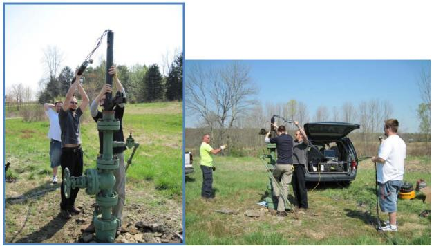
Figure 42 Launching the ILI tool into an observation well in North Canton, Ohio
