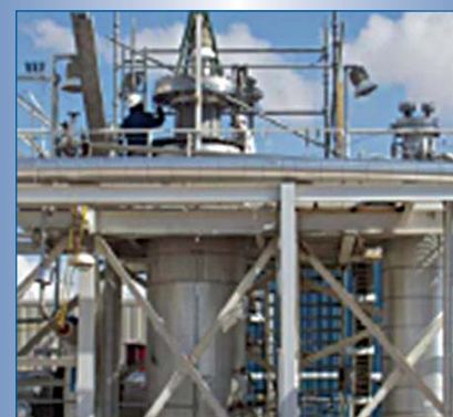
Figure 9. Nikkiso Cryo's liquefied natural gas pump undergoing tests.
