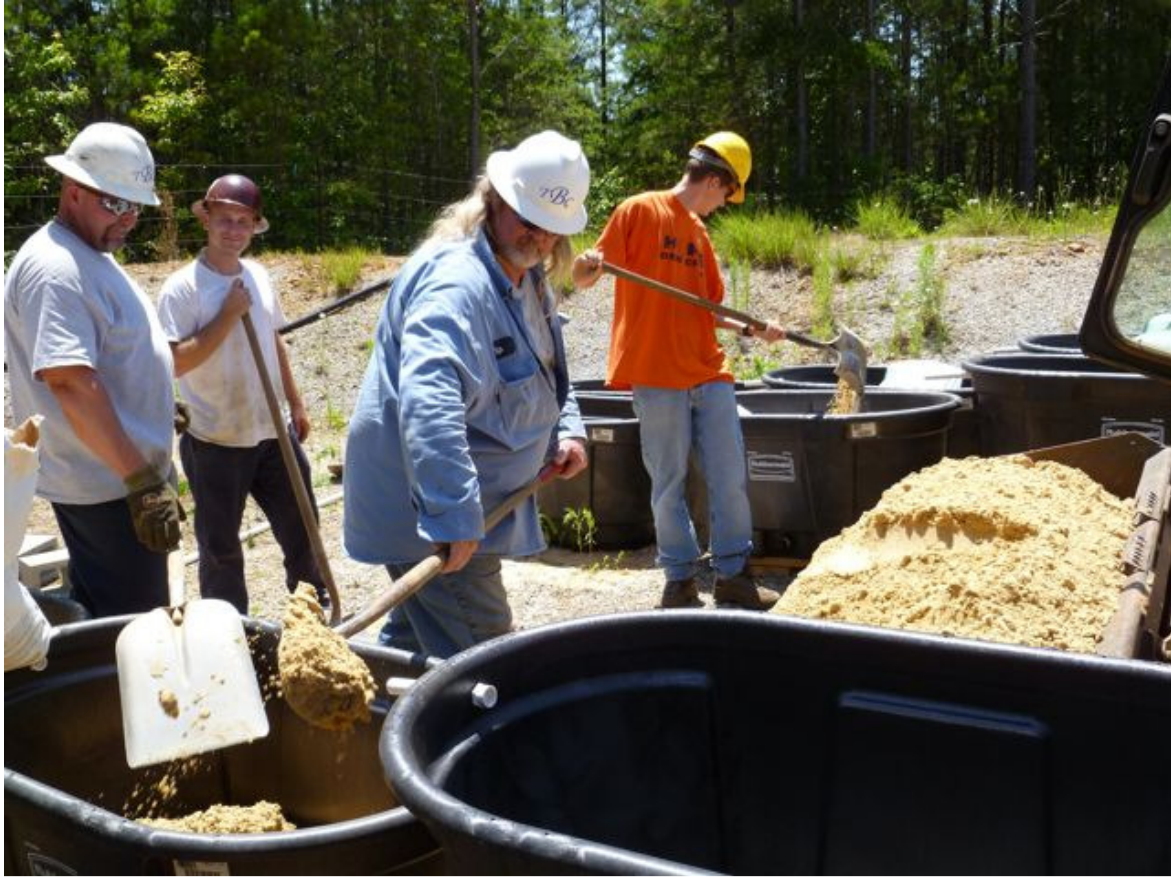
Figure 59. Filling the demonstration CWTS cells with sand.
