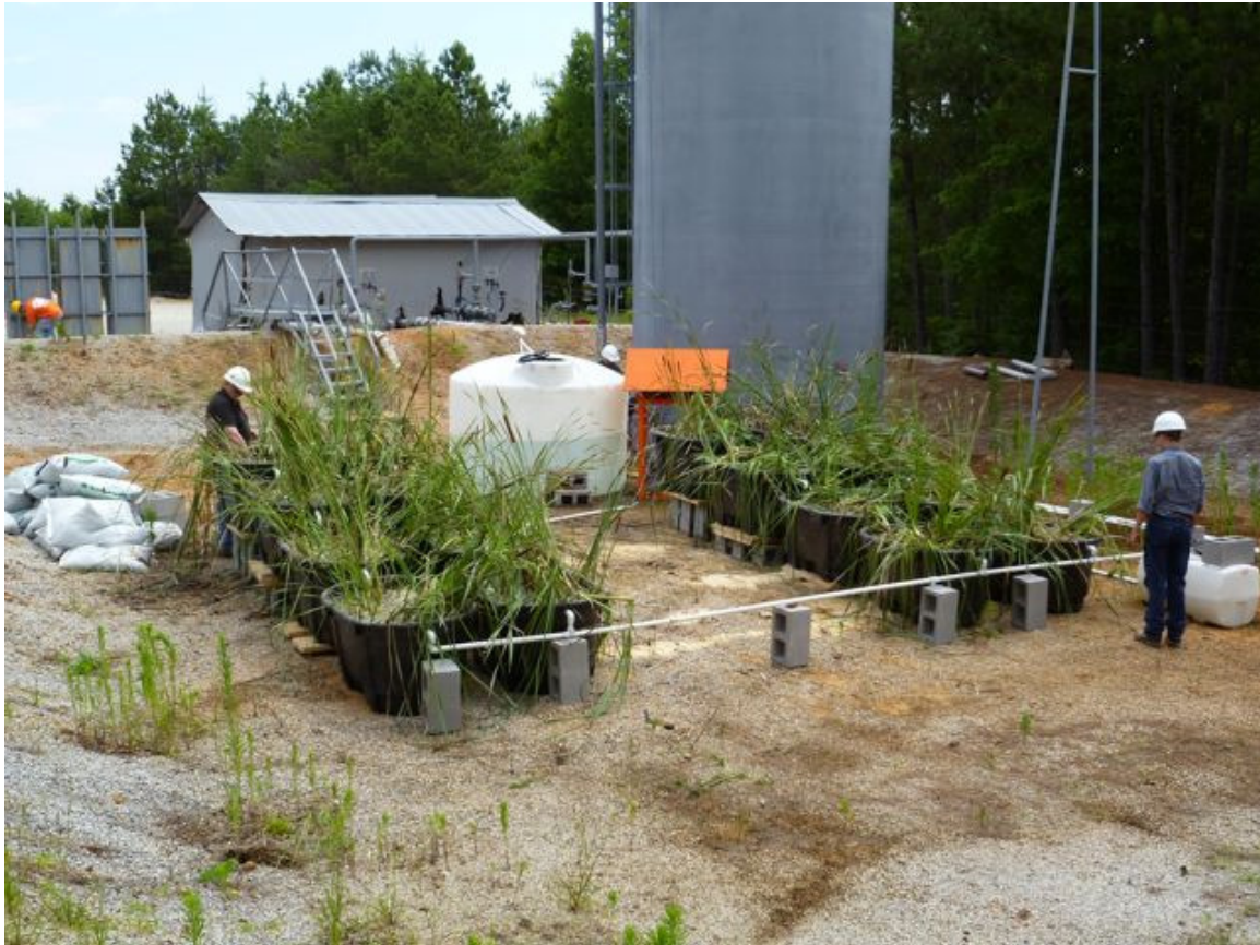
Figure 61. Demonstration CWTS after planting was completed on 5/31/12. Municipal water was introduced initially to the four series to allow growth and maturation of the plants and microbes.
