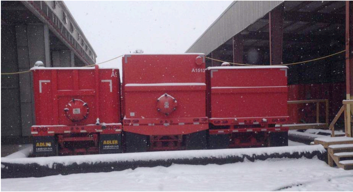
Figure 5.1 Frac tanks for flowback water and AMD storage
