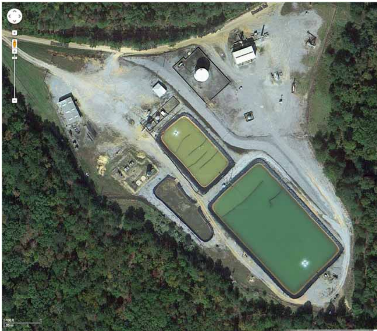
Figure 84.—Aerial photograph of two-stage water treatment facility in Robinson's Bend Field. Aerators and a system of baffles are used to facilitate evaporation of volatile compounds and to facilitate precipitation, flocculation, and suspension settling of particulate matter so that water can be discharged safely into the Black Warrior River.
