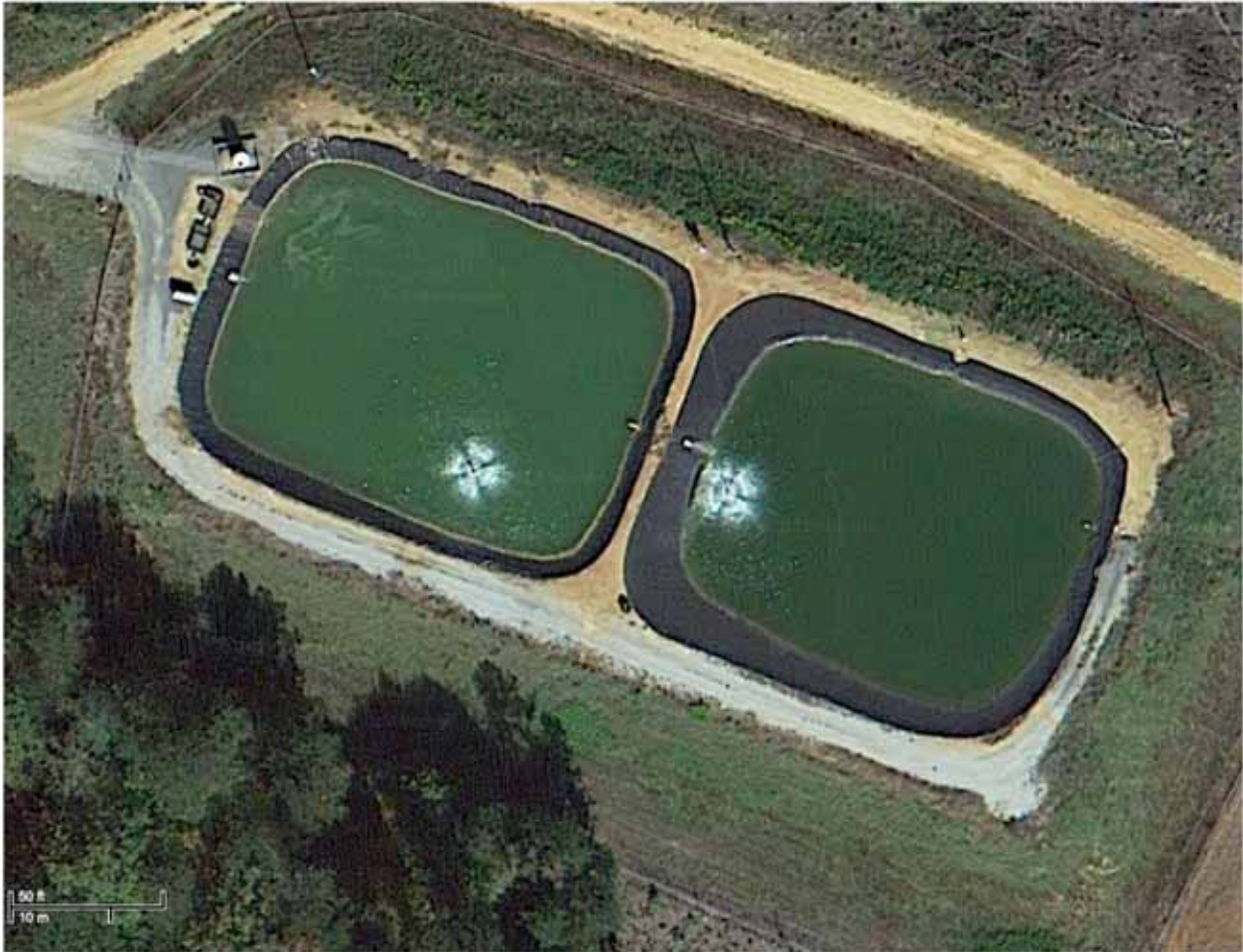
Figure 83.—Lined water treatment impoundments with aerators, which are widely deployed in the Black Warrior CBM fields to prepare produced water for discharge into streams.
