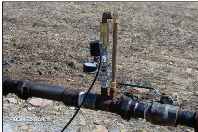
Figure 2. An FP-1 Sensor mounted in the flowline downstream of the wellhead.
