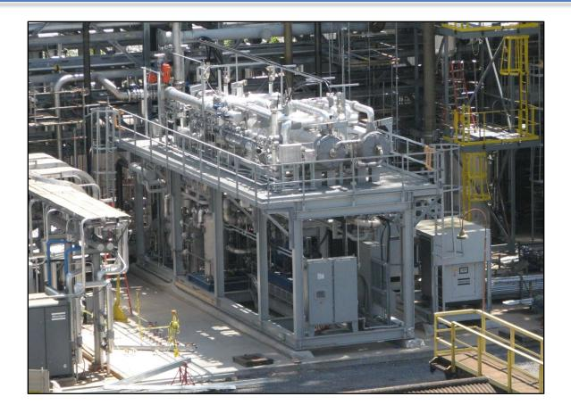
Data collected and lessons learned on MTR's 500 lb/hr flue gas bench-scale membrane used to support design and equipment selections of 10,000 lb/hr pilot-scale membrane.
