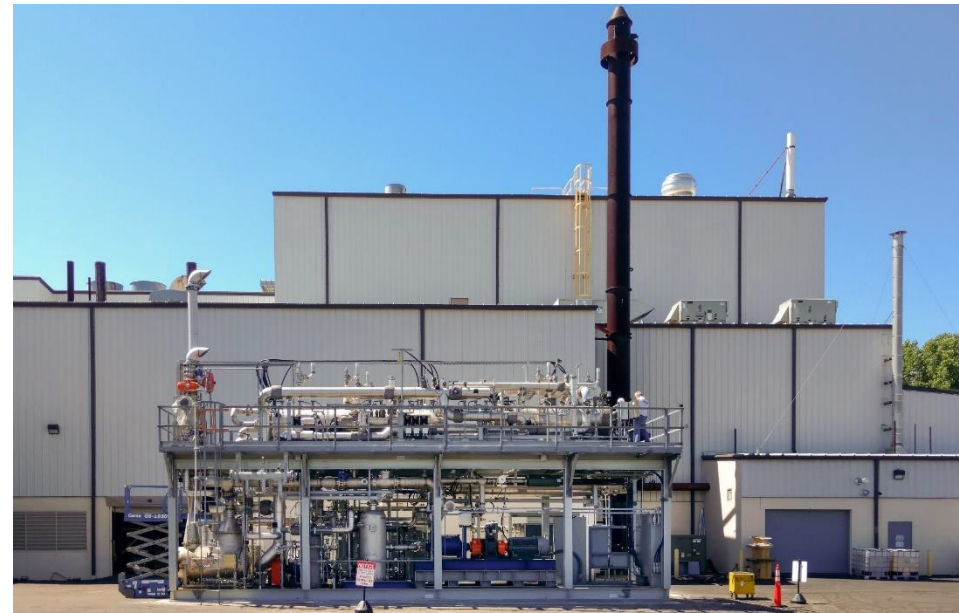
Main skid and smaller low-pressure drop sweep module anchored to foundation
