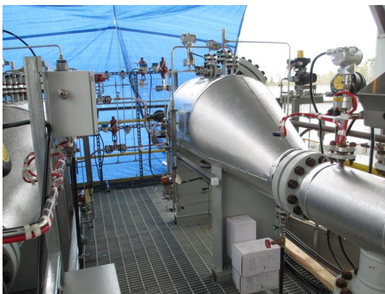
Figure 82. A photograph of skid B-1 with sulfur condensers.
