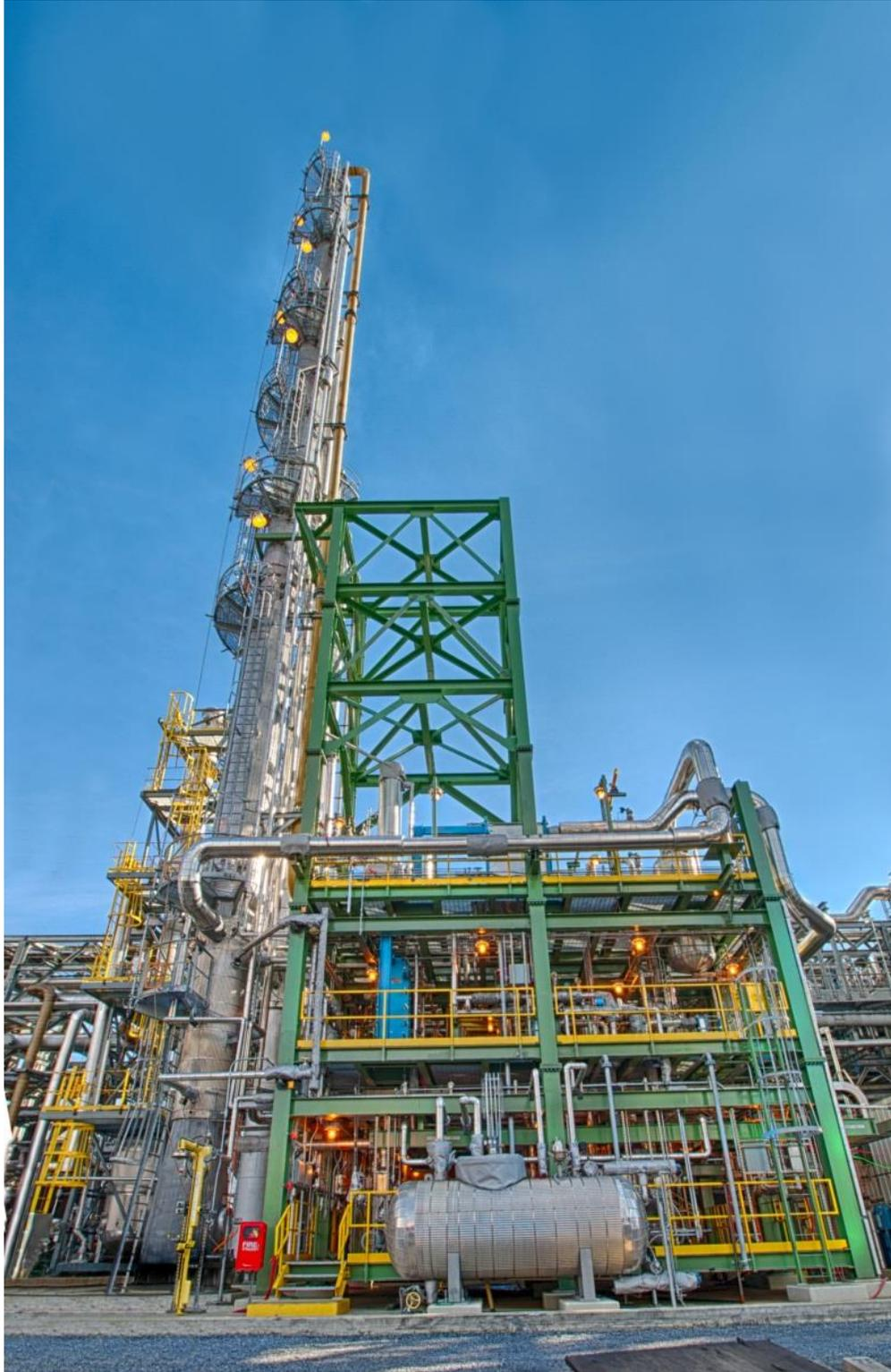
**Figure A-2: Linde-BASF 1-1.5 MWe PCC pilot plant installed and tested at NCCC**
