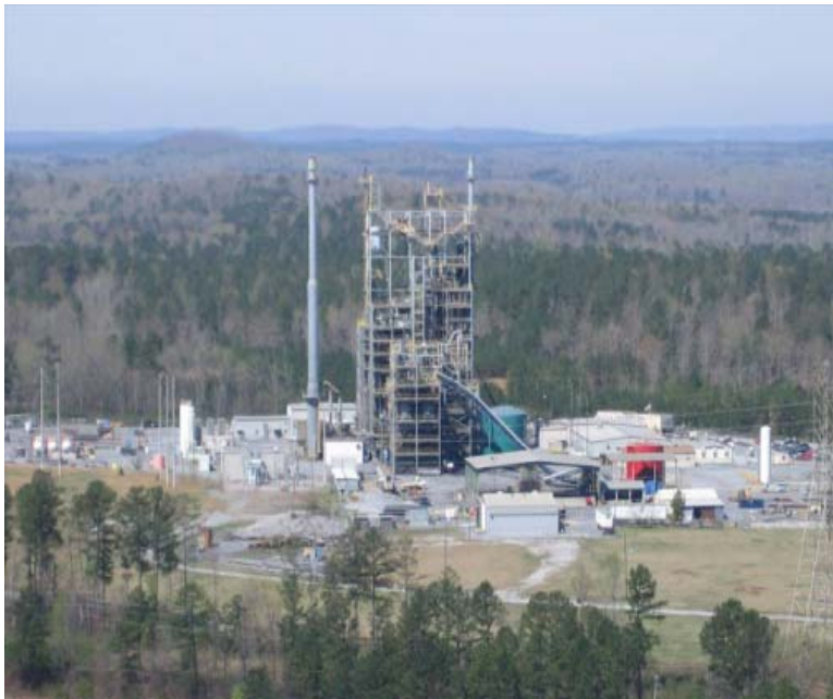
Pre-combustion CO2 capture facility
