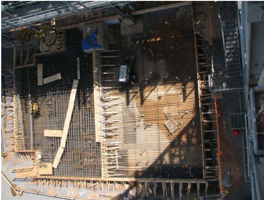
Rebar Placement
