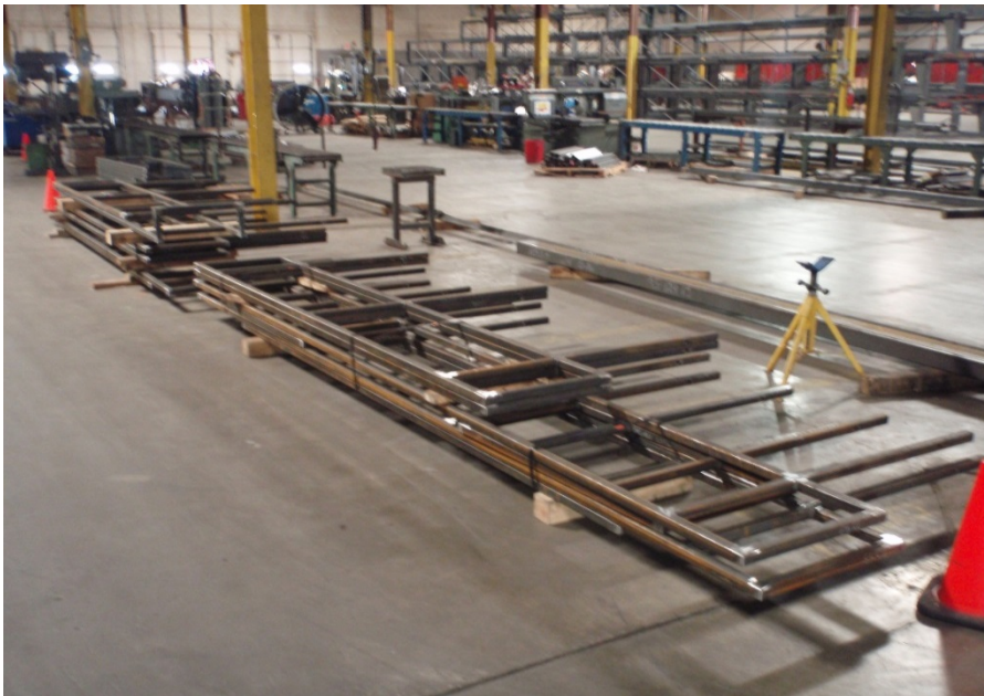
Steel structures in shop fabrication
