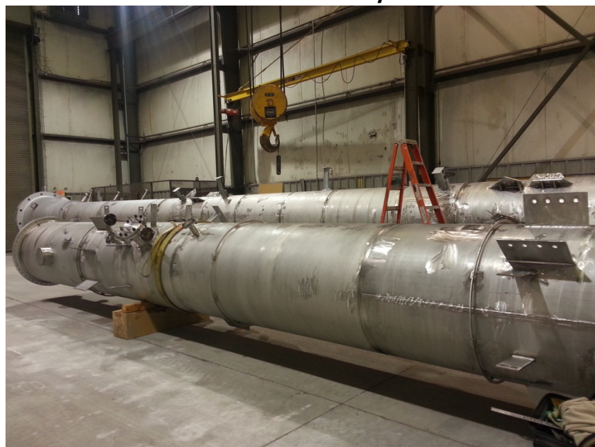
Absorber section in fabrication and assembly
