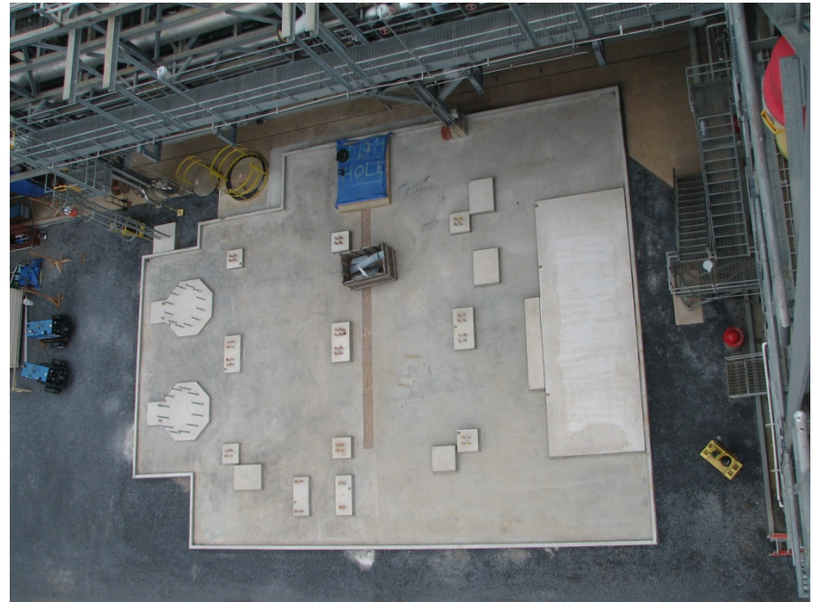
Foundations and Slab Complete
