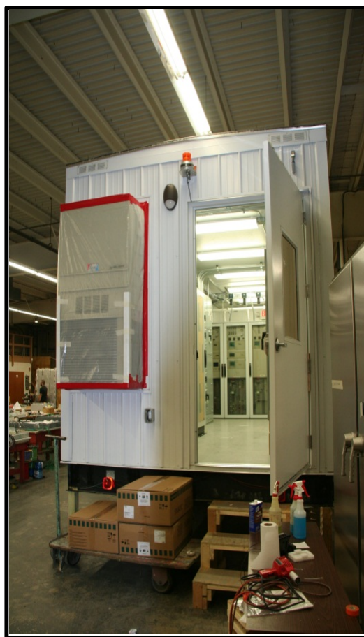
Analyzer and controls container
