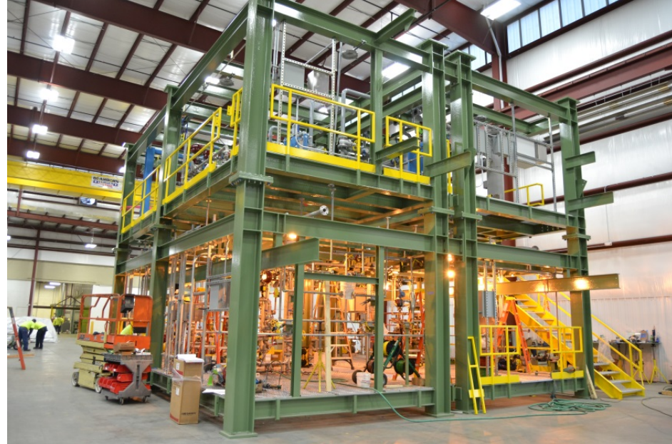
Module installation & Assembly
