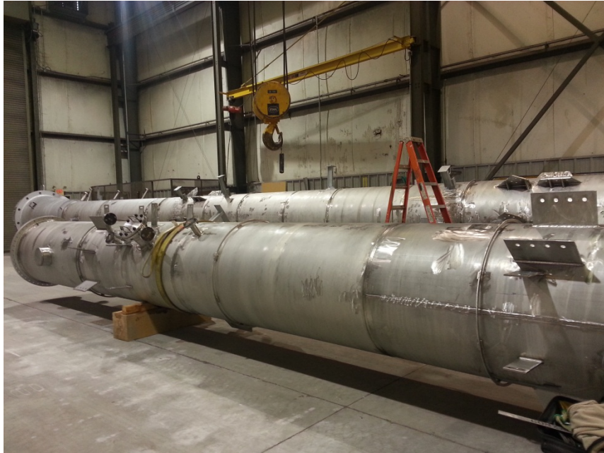
Absorber section in fabrication and assembly
