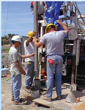
UNAVCO Installing Borehole Strainmeter
