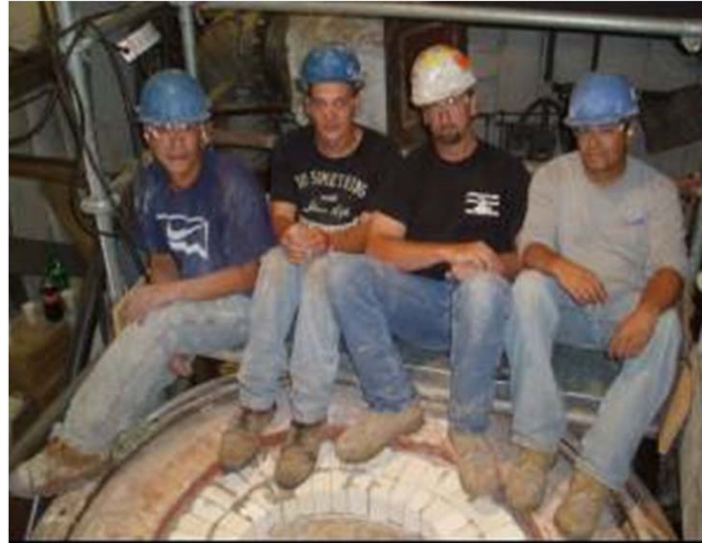
Top of oxidizer after refrax liner installed
