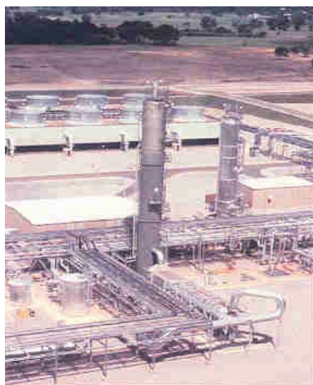
Picture 3: Absorber (foreground) and stripper (background) 1
