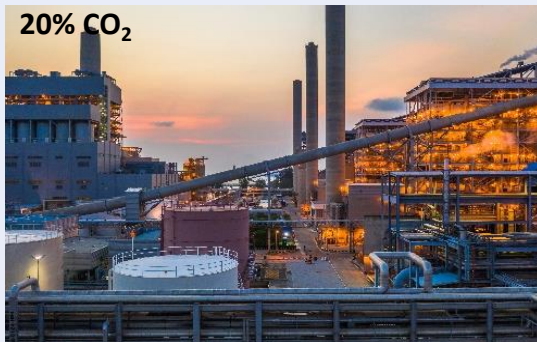
Iron and Steel Plants
