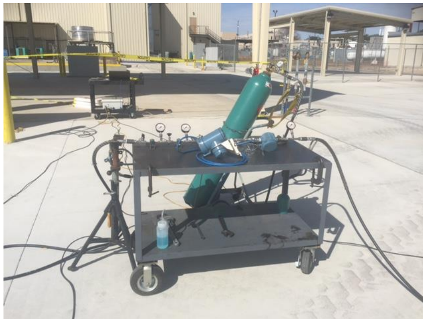
Figure 5: Methane Tank with Release Valves
