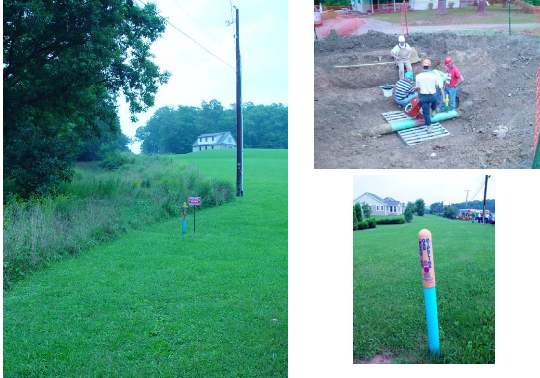
Figure LXXIV :Site of live test-site
