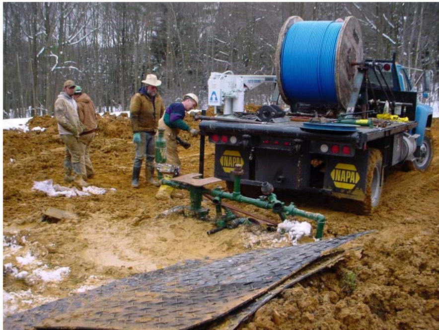
Figure 15 – Rigging-up Flexible Tubing Spool
