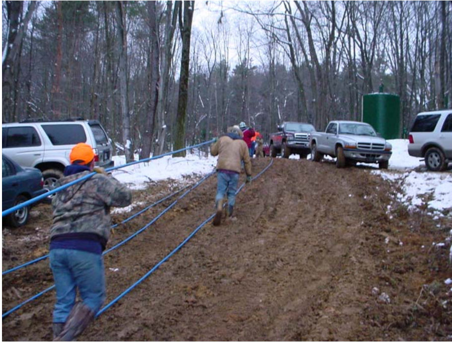
Figure 17 – Laying Down the Velocity String
