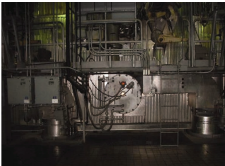
2. Eye on optimization. Cyclone boilers pose unique optimization challenges. CombustionOpt successfully managed cyclone stoichiometries toward steady operation. Such management of stoichiometries is instrumental in avoiding slugging. Courtesy: Dynegy Inc.
