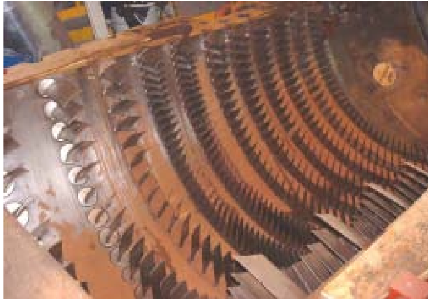
Fig. 3. Axial Flow Compressor Stators located in the casing
