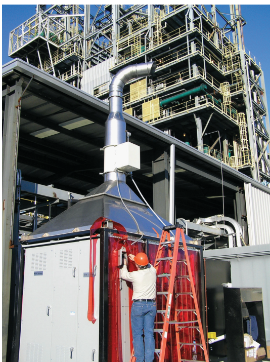
NETL researcher Rich Pineault installs the SOFC multi-cell array at the PSDF gasification facility in Alabama, with the gasifier visible in the background
