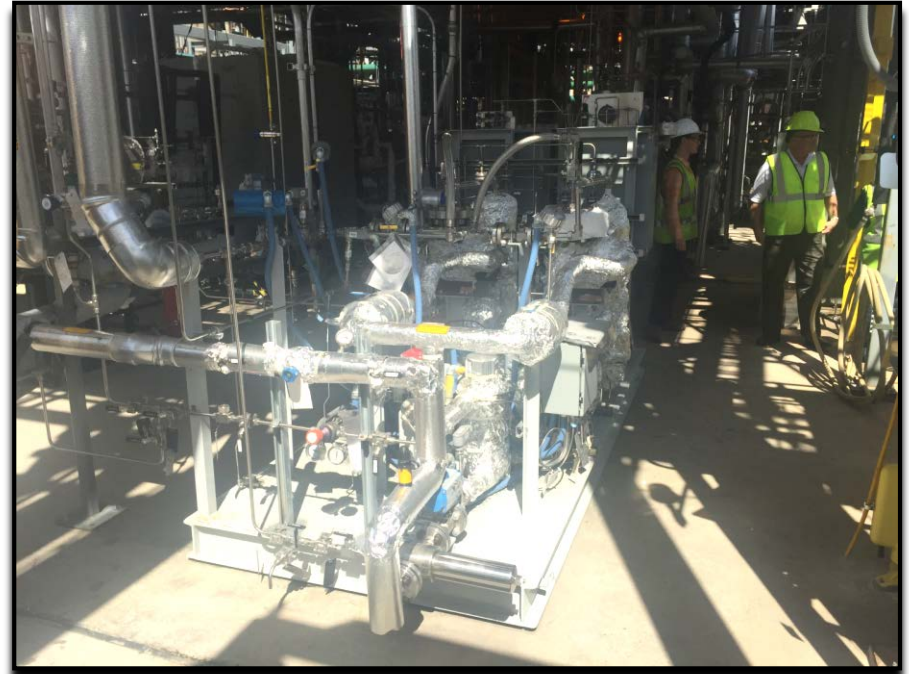
Photograph of the skid installed at the NCCC (April 2017)
